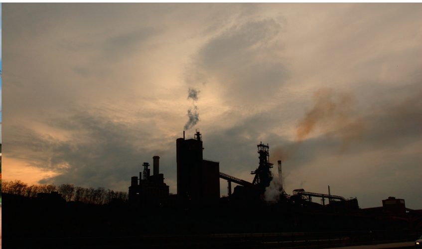
Cockerill-Sambre is a Belgian steel manufacturer located in Seraing Photo: Luc Viatour ( https://Lucnix.be )
